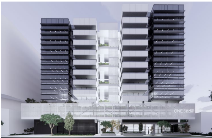
Image 2. Photomontage of now completed development at 1-5 Chalmers Crescent. Site no. 7 from figure 1.
